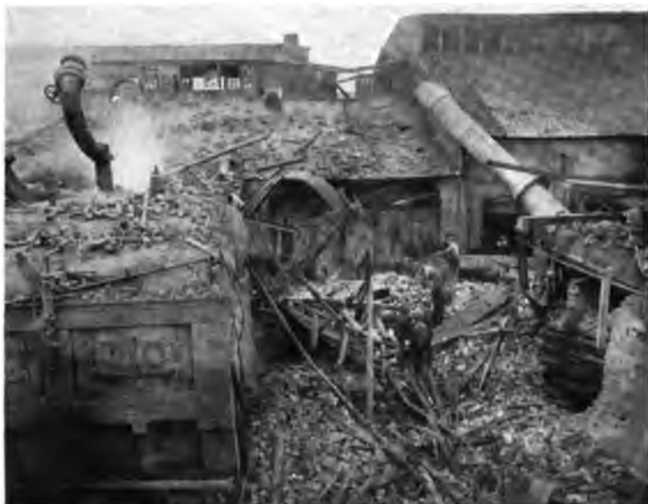
Fig. 3. Plant wrecked by Boiler Explosion.
